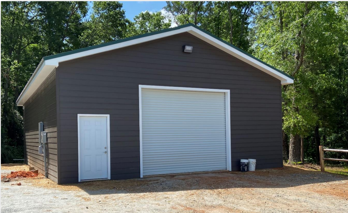
New Maintenance Building at Ellerslie Park (Constructed by Facilities Maintenance and Inmate Crews)
