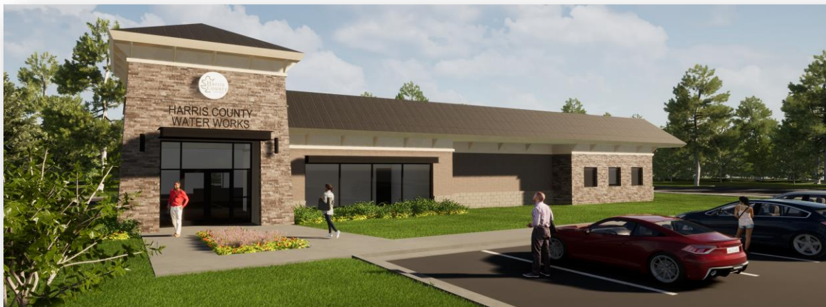
New Water Works Administration Building
