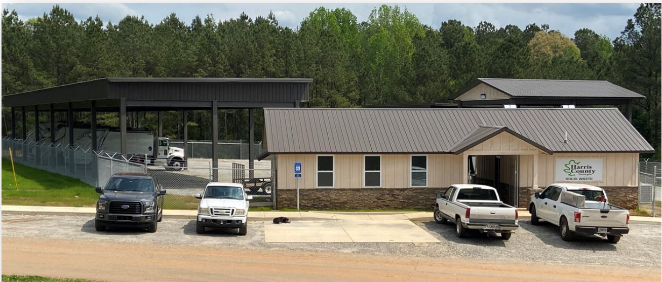
New Solid Waste Facility
