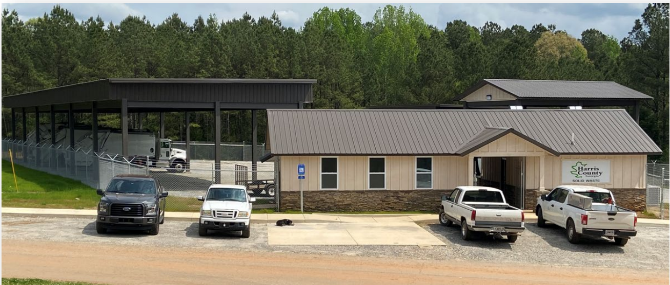
New Solid Waste Facility
