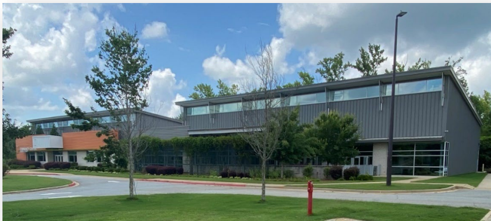
Harris County's Community Center
