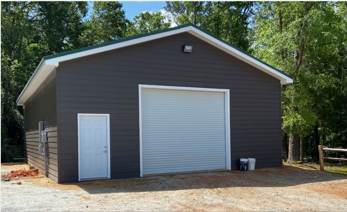
New Maintenance Building at Ellerslie Park (Constructed by Facilities Maintenance and Inmate Crews)
