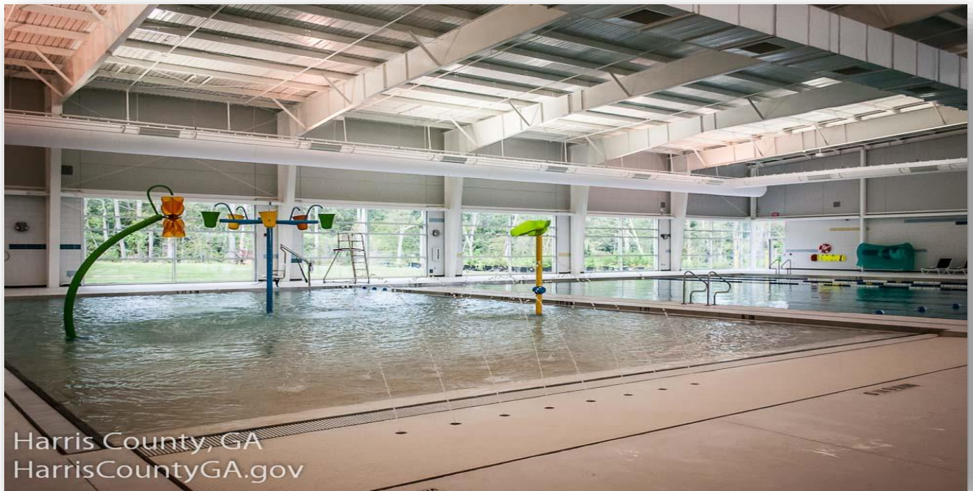
Community Center's 25 meter eight lane competition pool and children's zero-entry leisure area
