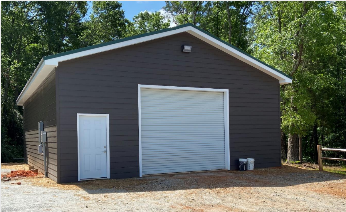
New Maintenance Building at Eilerslie Park (Constructed by Facilities Maintenance and Inmate Crews)
