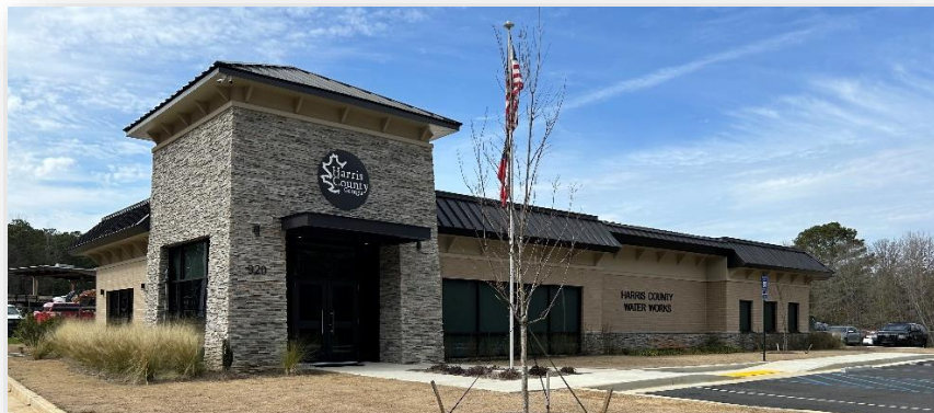
New Water Works Administration Building
